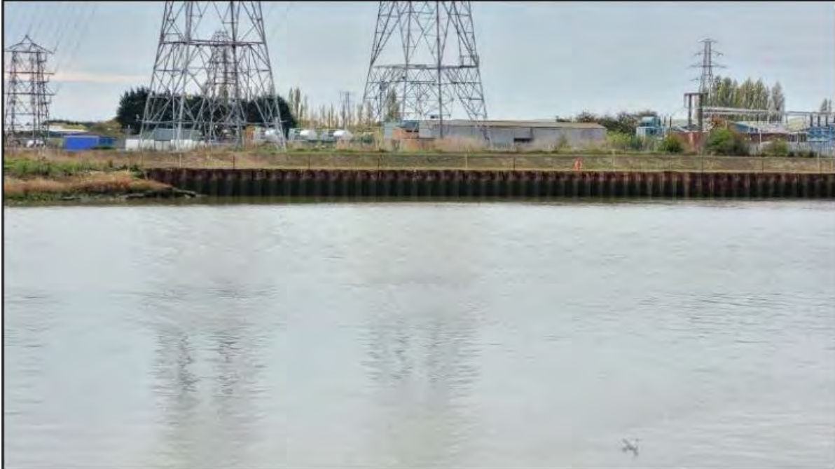
Figure 2 Ground view of securable land behind sheet-pile wall in south bank of The Haven (credit: Andrew Chick Ecology)
