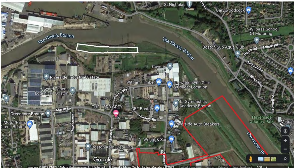
Figure 3 Annotated aerial view showing the indicative outline of raised land (within white polygon) behind sheet-pile wall in the bank, opposite Port of Boston lock on north side of The Haven. Principal Application Site lies within red line. (Imagery copyright 2022 Google, CNES / Airbus, Getmapping plc, Infoterra Ltd & Bluesky, Maxar Technologies, Map data copyright 2022)
